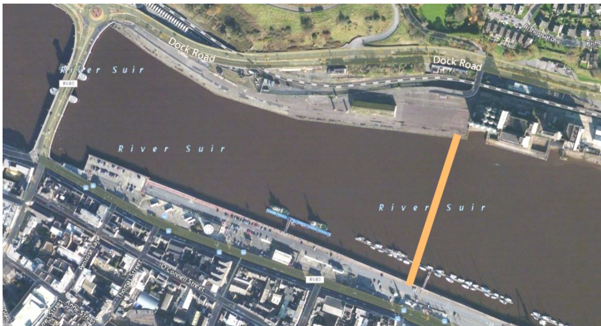
Figure 1. Location of proposed bridge in Waterford City
